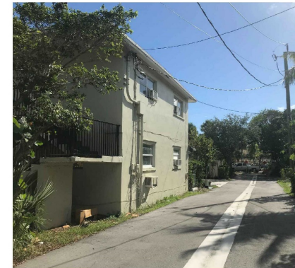
1 EXISTING PARTIAL NORTHWEST CORNER
