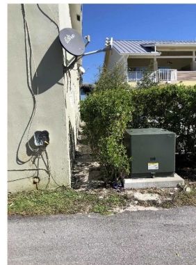
6 EXISTING SOUTHWEST CORNER
