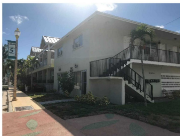
10 EXISTING NORTHEAST CORNER
