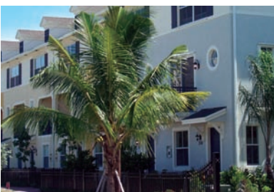
Atlantic Grove, on West Atlantic Avenue, was a mixed-use project that included ten affordable townhouses.
