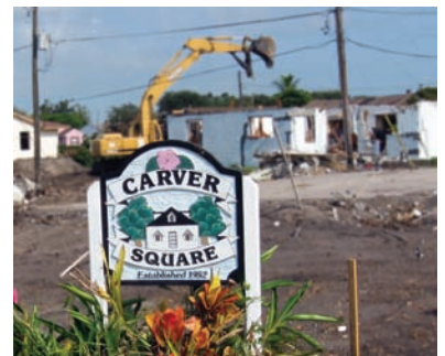
The CRA purchased the structurally damaged homes in Carver Square and provided residents with funds for relocation.
